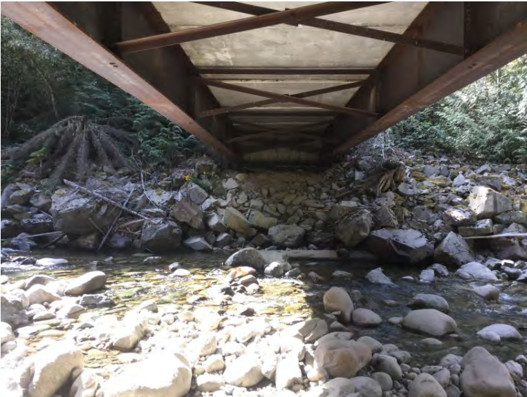
Left Bank Abutment when facing downstream
