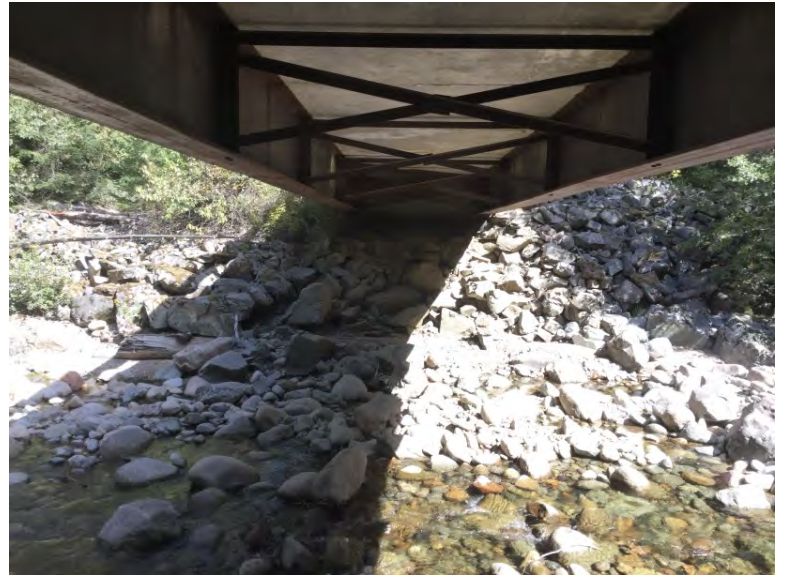
Right Bank Abutment when facing downstream
