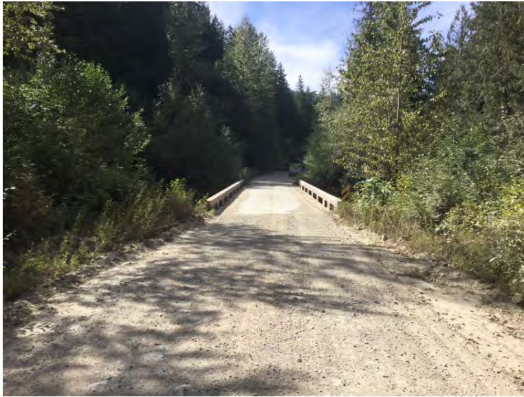
Approach from Right Bank when facing downstream
